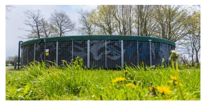
The mesh silo is designed to provide extra storage of slurry or water, is quick to install and relocateable. The mesh silo can be used for the storage of various liquids including slurry, clean and dirty water.
