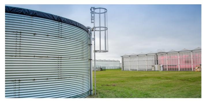
The Genap silo- and cage ladders are a robust system for safe inspection of the contents of a water silo. A major advantage of this ladder is that the mounting brackets can be attached without altering or loosening the existing silo bolts. This avoids entering the tank or partially removing the lining.
