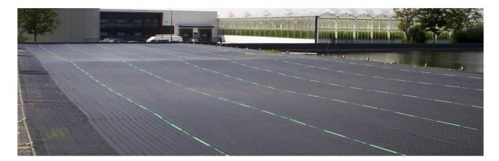
When water is stored in a water reservoir without a cover, algae growth and other types of contaminations generally have free reign. As a result, irrigation systems are likely to get blocked, causing all kinds of undesired consequences. An anti-algae water reservoir cover prevents contamination and keeps the water permanently clean. In addition, the storage capacity of the water reservoir is maximized, as the cover reduces wave formation and evaporation.
