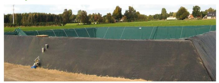
The Genap slurry reservoir is a Kiwa certified excavated reservoir designed for the storage of various types of liquid slurry and digestate. The reservoir is excavated and lined with a membrane, and the soil excavated is used to construct the embankments around the reservoir. You can order a slurry reservoir in any size; we customize it to your needs.
