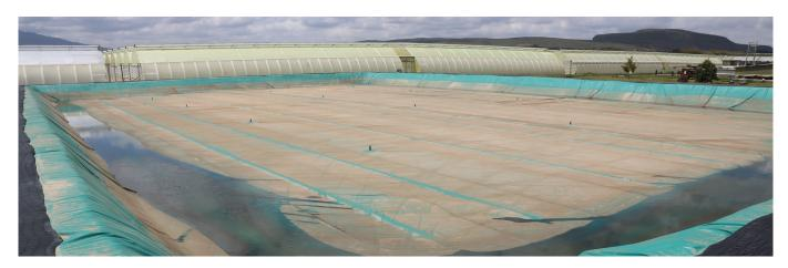
In countries that suffer extreme temperatures, a fully closed water reservoir is increasingly chosen for the storage of irrigation water. This minimises the external influences on water quality. Such a system is the best solution against algae growth or contamination due to sand or other dirt. But wave formation and evaporation are also prevented for maximum utilisation of the storage capacity.
