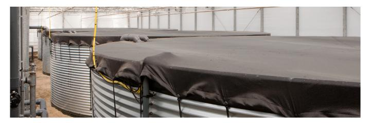
When water is stored in a silo without a cover, algae growth, wind borne debris entering the silo and evaporation can occur. As a result, irrigation systems can get blocked reducing the efficiency and effectiveness of the system. An anti-algae tensioned silo cover prevents the growth of algae and keeps the water free of contamination. In addition, the cover maximizes the storage capacity of the silo, reduces wave formation and prevents evaporation.
