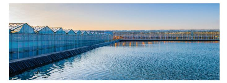
A dug and embanked pond is a good way of storing very large volumes of water in a manageable way. The Genap pond is specially designed for direct collection of rainwater via pumping systems, greenhouse roofs, buffer wells and gutters.
