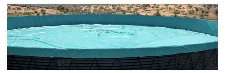
The GenaFlexstore® is a worldwide patented fully closed water storage system in which the flexible silo liner and floating cover are integrated into one system. This means that it is virtually impossible for external factors to influence the quality of the water. The GenaFlexstore® is completely closed and with almost no evaporation possible the capacity of the silo can be fully utilized.
