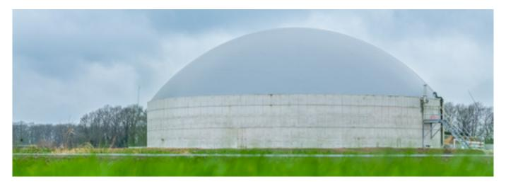
Biogas is a future-proof energy source, generated from organic waste streams and slurry. For the digester silos in which biogas is produced and stored, Genap has developed the 'Double Membrane Biogas cover'.
