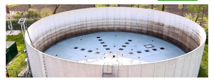
The Biogas floating cover is a floating cover system for collecting biogas from digestate that Genap developed in cooperation with N-E-ST based in Ahaus, Germany.
