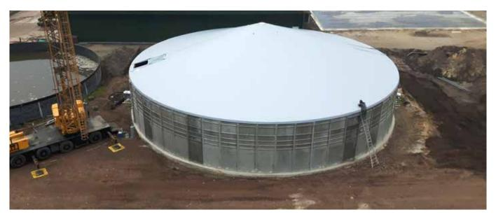
The Genap tensioned cover is designed specifically to serve as an emission-reducing cover and is perfect for covering a silo made of concrete, steel or wood. This made-to-measure cover is robust, maintenance-free, durable and resistant to slurry and other aggressive liquids. The tension cover includes a statistical calculation based on the desired application and the climatic conditions at site.
