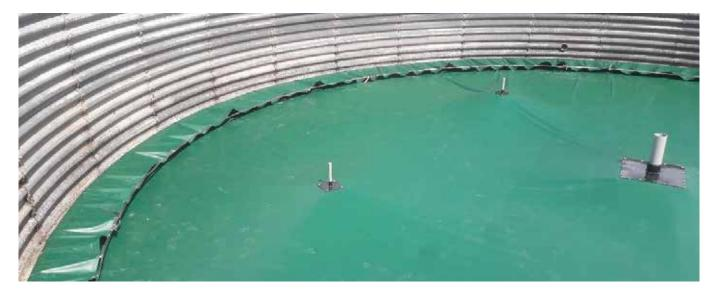
For silo constructions that cannot support a tensioned cover, a floating cover is an excellent alternative. The made-to-measure cover floats on the slurry and goes up and down with the slurry volume. Rainwater collected on the cover can be pumped off to prevent it from mixing with the slurry, allowing optimum use of the storage system.
